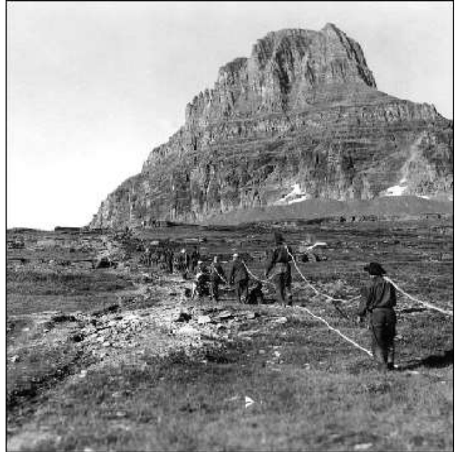
CCC workers carry the trans-mountain telephone cable from Logan Pass towards Hidden Lake Pass.
